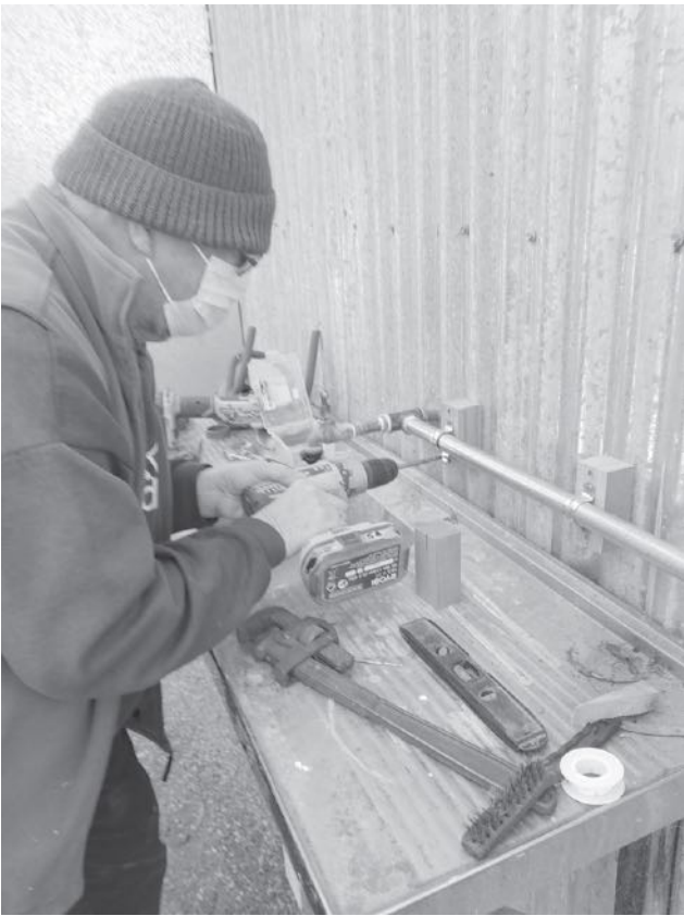
☆ Alan, in the process of completing the pipe work for the garden bed watering system.
