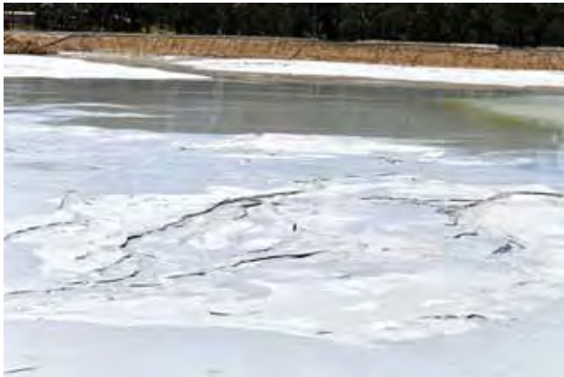
☆ Tailings (remains of the ore) in a large purpose built dam on site.
