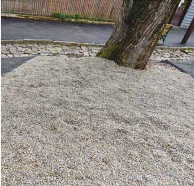
☆ Trial infill material for tree bases - crushed granite.
