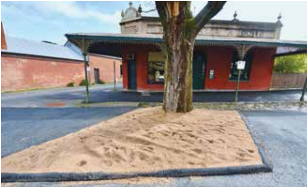
☆ Trial infill material for tree bases - granite sand.
